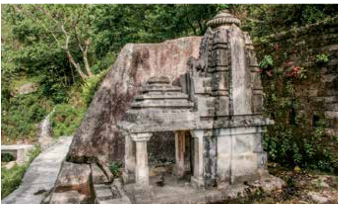
Monolithic rock-cut shrine and water structure, ca. 850–1000, Almiya, Uttarakhand
